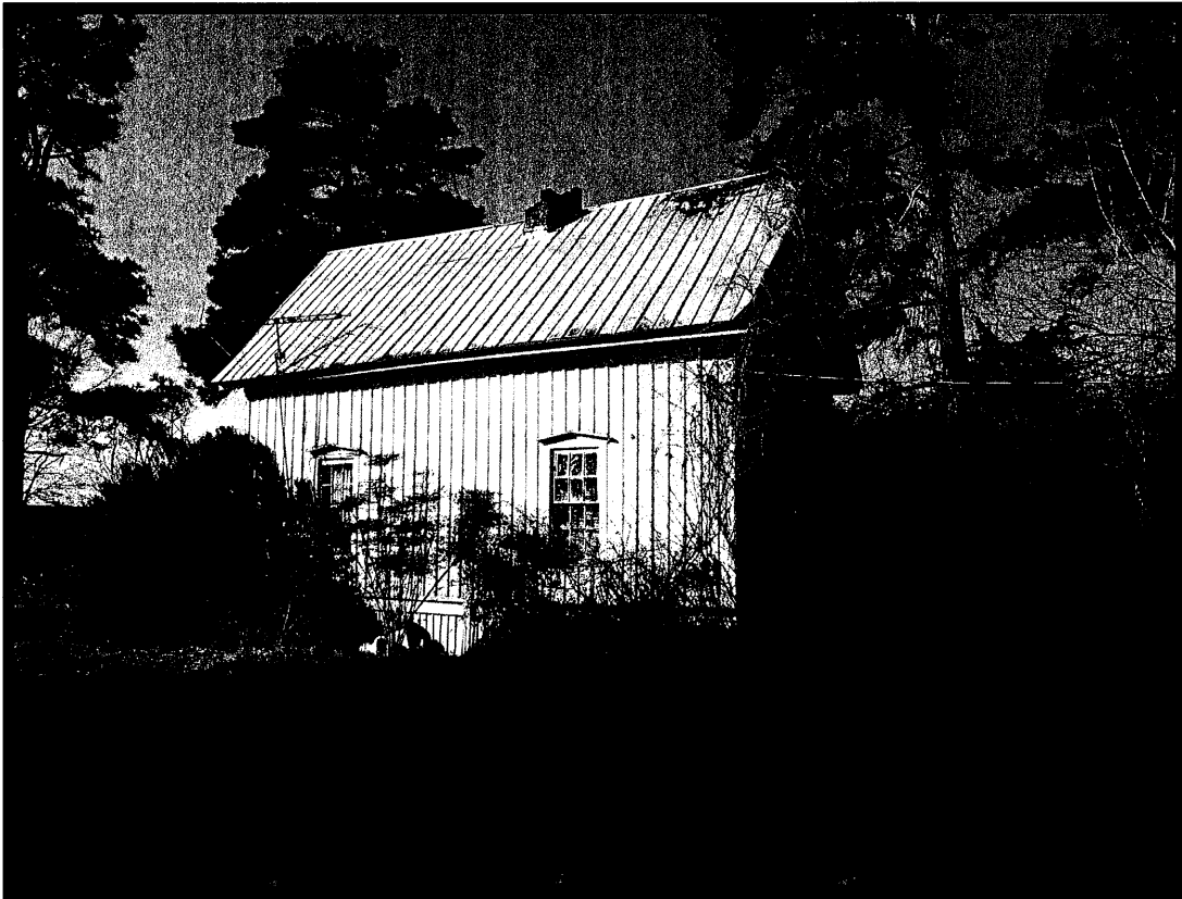
Figure 5.3-4: View of Nat Dunn House, Looking Southwest.
