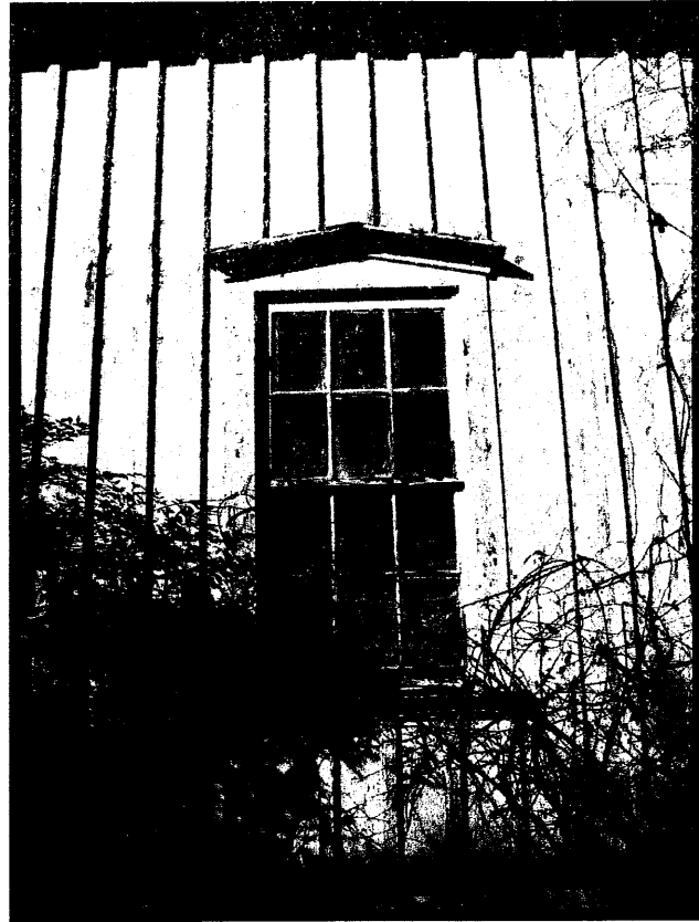
Figure 5.3-7: View of Nat Dunn House, Detail of Window and Siding.
